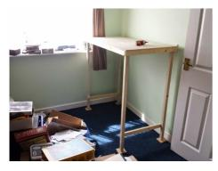
With all the tables installed it gives me an 11 foot run down the left wall with 6' 6" x 2' wide and the remaining 4' 6" x 3' 3" wide. Underneath the window is a 2' 6" x 2' board which is finally joined to the the 4' x 2' board by the door.
